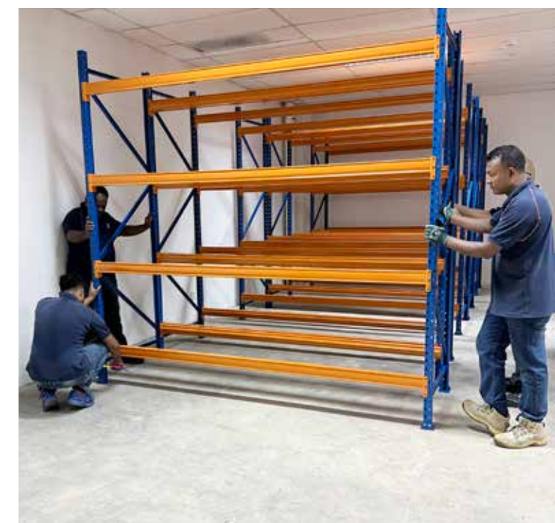
Improvement works for the SAFM artefact store.
